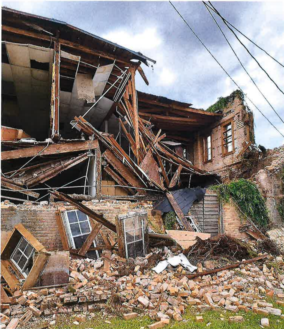
Photograph #1: View of building failure showing collapsed walls, second floor and roof.
