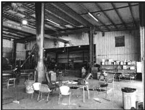
View of fabrication area (facing S)
