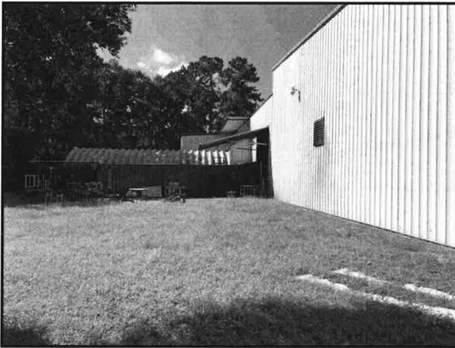
View, facing S, of rear building elevation (quonset and container storage portions in distance).
