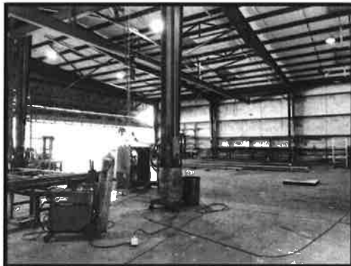
View, facing N, of NLY fabrication area
